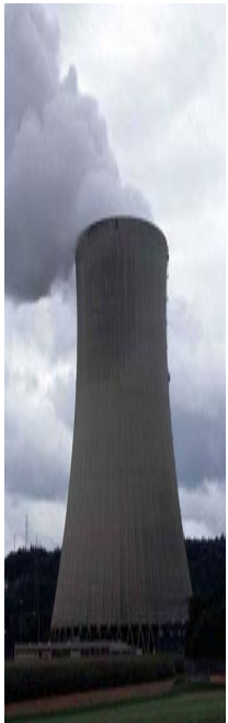
Arkansas's one nuclear power plant on Lake Dardanelle
